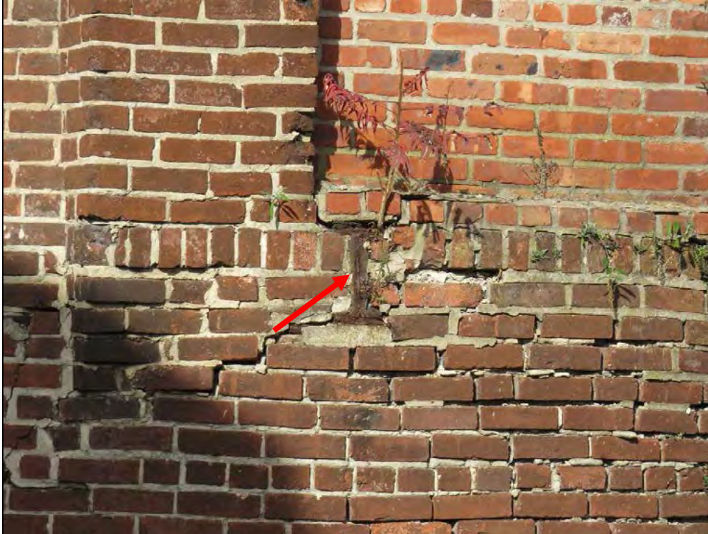
Photograph 25: The embedded steel beams still remaining are heavily corroded and causing displacement of the surrounding masonry.
