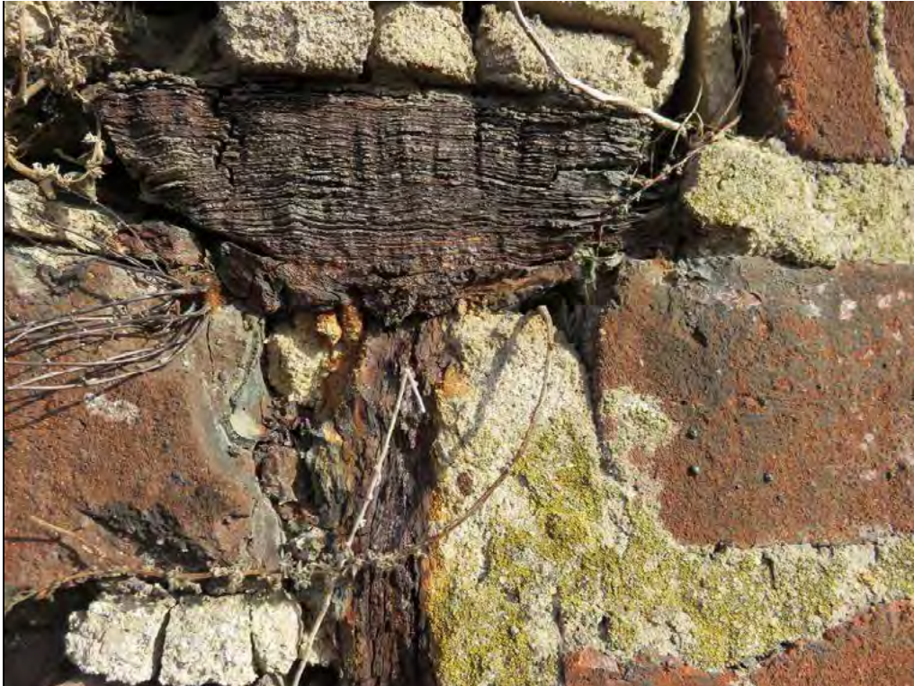
Photograph 27: The expansion of the steel as it corrodes puts stress on the surrounding masonry. This steel beam has expanded to be multiple times larger than it was originally.
