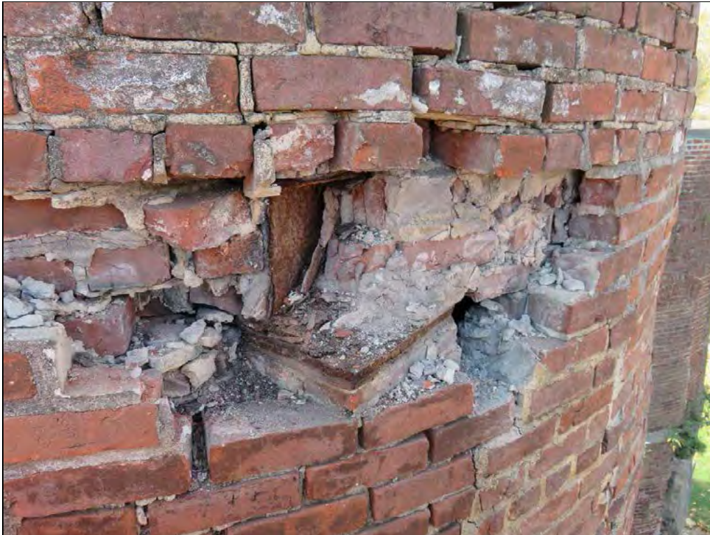
Photograph 26: The embedded steel beam was heavily corroded.
