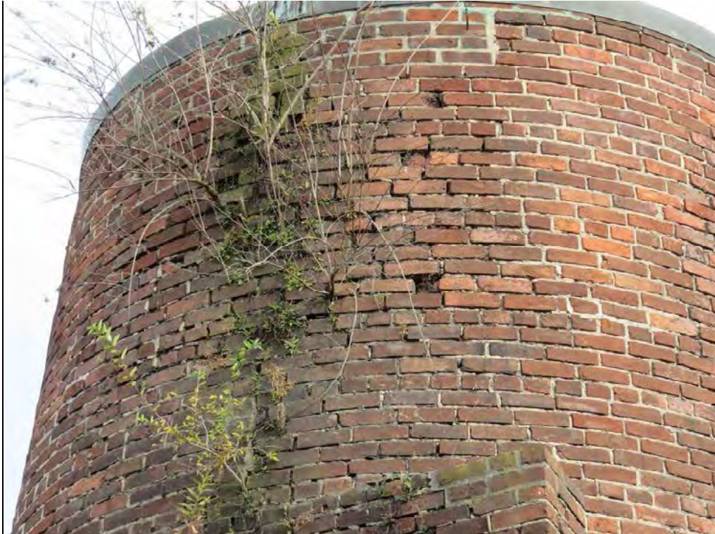
Photograph 23: As the plants get bigger the masonry deterioration surrounding the areas increases.
