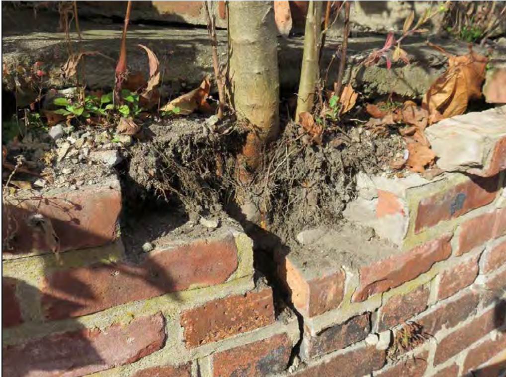
Photograph 24: Eventually the roots get large enough to cause displacement of the surrounding masonry.
