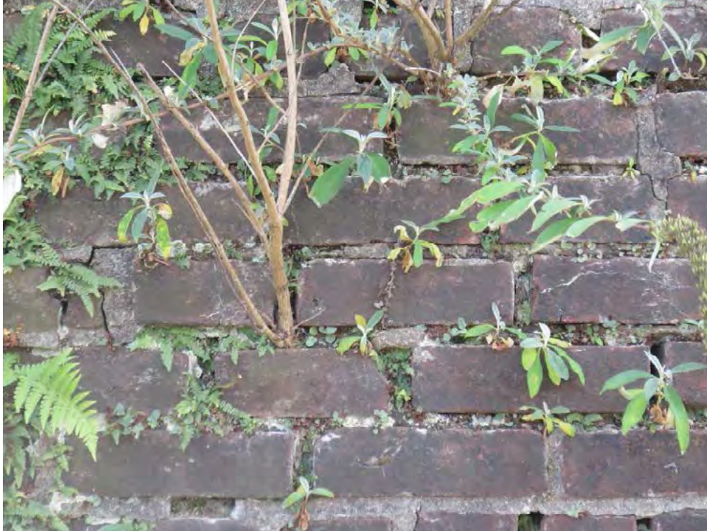
Photograph 22: The roots of the plants take hold in the missing mortar joints and expand as they grow.
