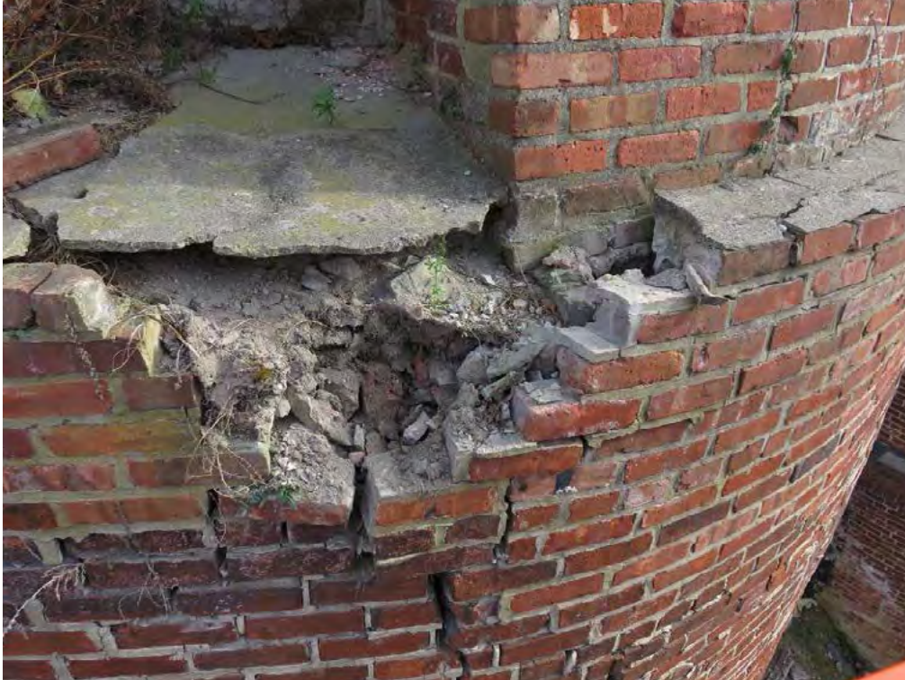
Photograph 16: The loss of the brick veneer creates large openings for bulk rain water to enter the wall assembly, increasing the rate of deterioration.
