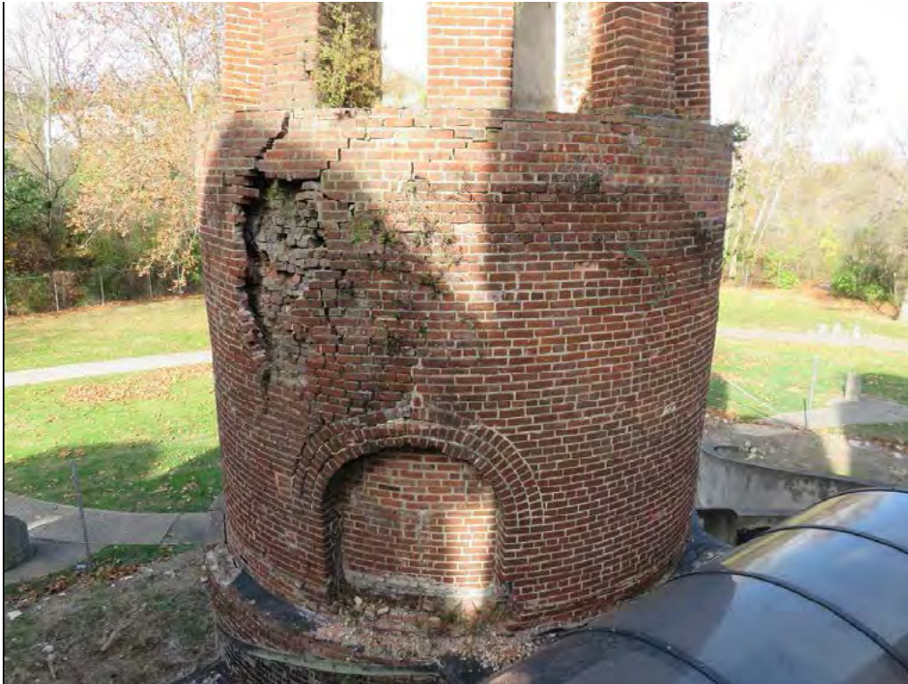
Photograph 17: Complete failure of the brick veneer.
